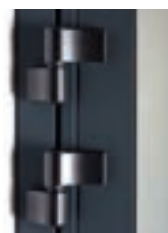
Paumelles et joint anti-pince doigts
